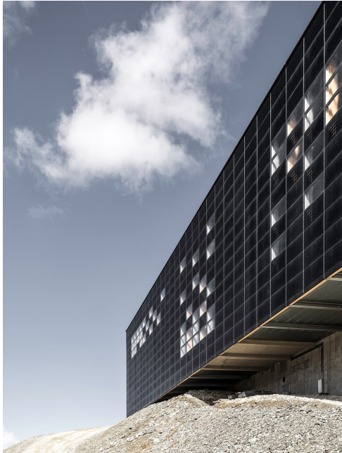
3S cableway station building facade. Source: Zermatt Bergbahnen
