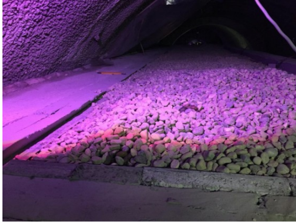
A look into the sensible thermal storage system at the pilot plant in Biasca. The storage solution is filled with pebbles with a diameter of around 2 centimetres. Source: Andreas Haselbacher
