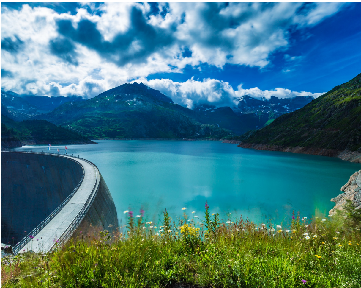
A dam in an idyllic landscape: Lac d'Emosson in the Valais Alps. Source: Adobe Stock
