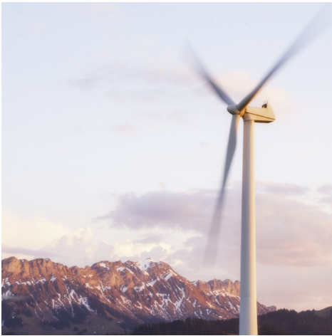
Real-time control of power flows
