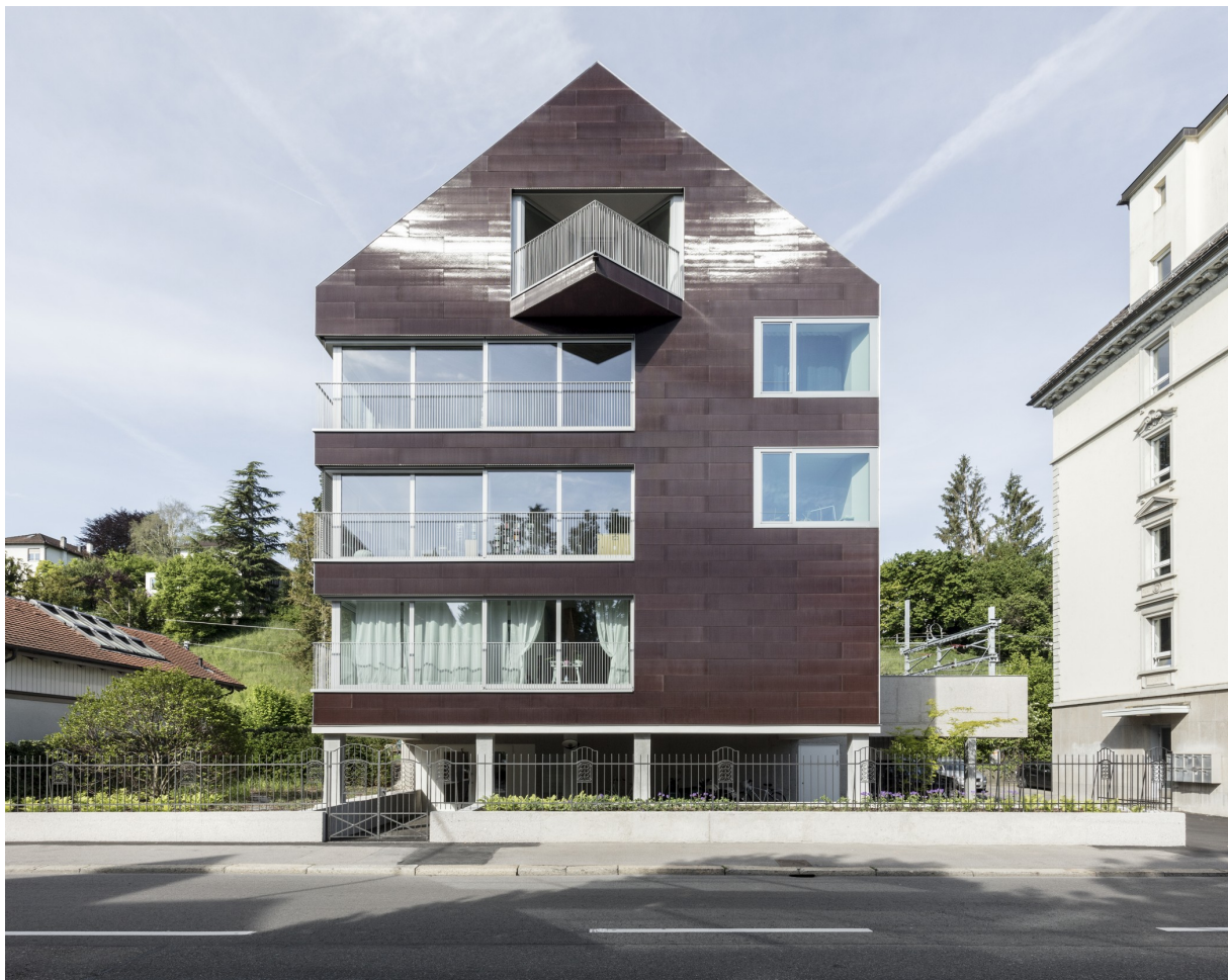
The colour-printed photovoltaic cells on the face of the "Solaris" residential building in Zurich cover the tenants' electricity needs. Source: Beat Bühler
