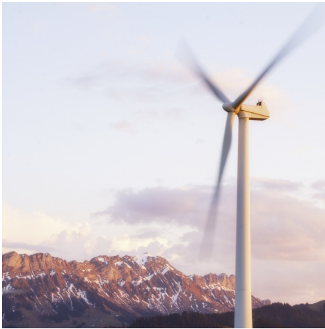
Real-time control of power flows
