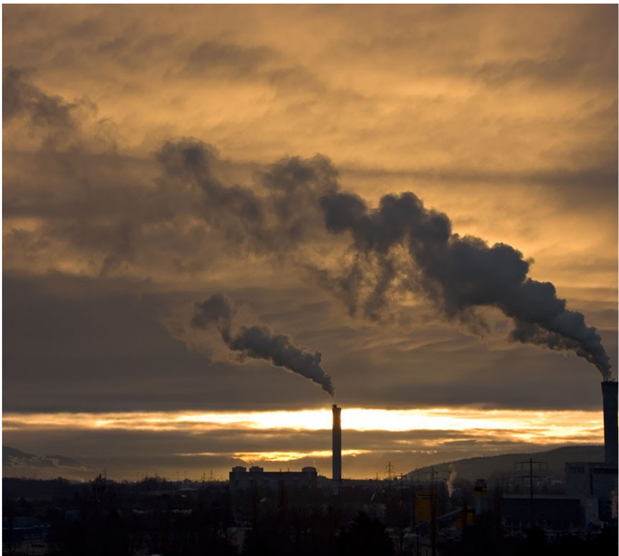
The Hagenholz waste incineration plant in Zurich (right), together with the Aubrugg wood-fired power plant (left), supplies most of Zurich's district heating grid. However, a lot of heat energy is still lost elsewhere. This could be utilised with the help of adsorption heat pumps. Source: Wikimedia/Marc Forster
