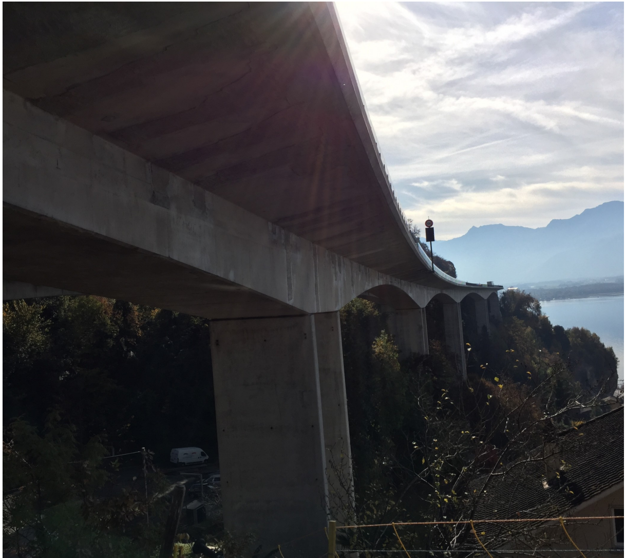
The Chillon Bridge was renovated with ultra-high-performance fibre reinforced concrete. Source: Eleni Chatzi
