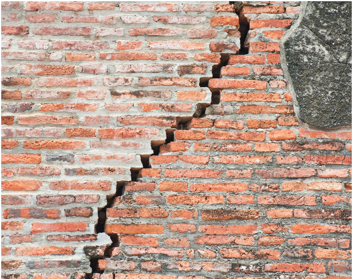
Damage such as cracks in walls should not occur – even if geothermal drilling is carried out nearby. Source: Shutterstock
