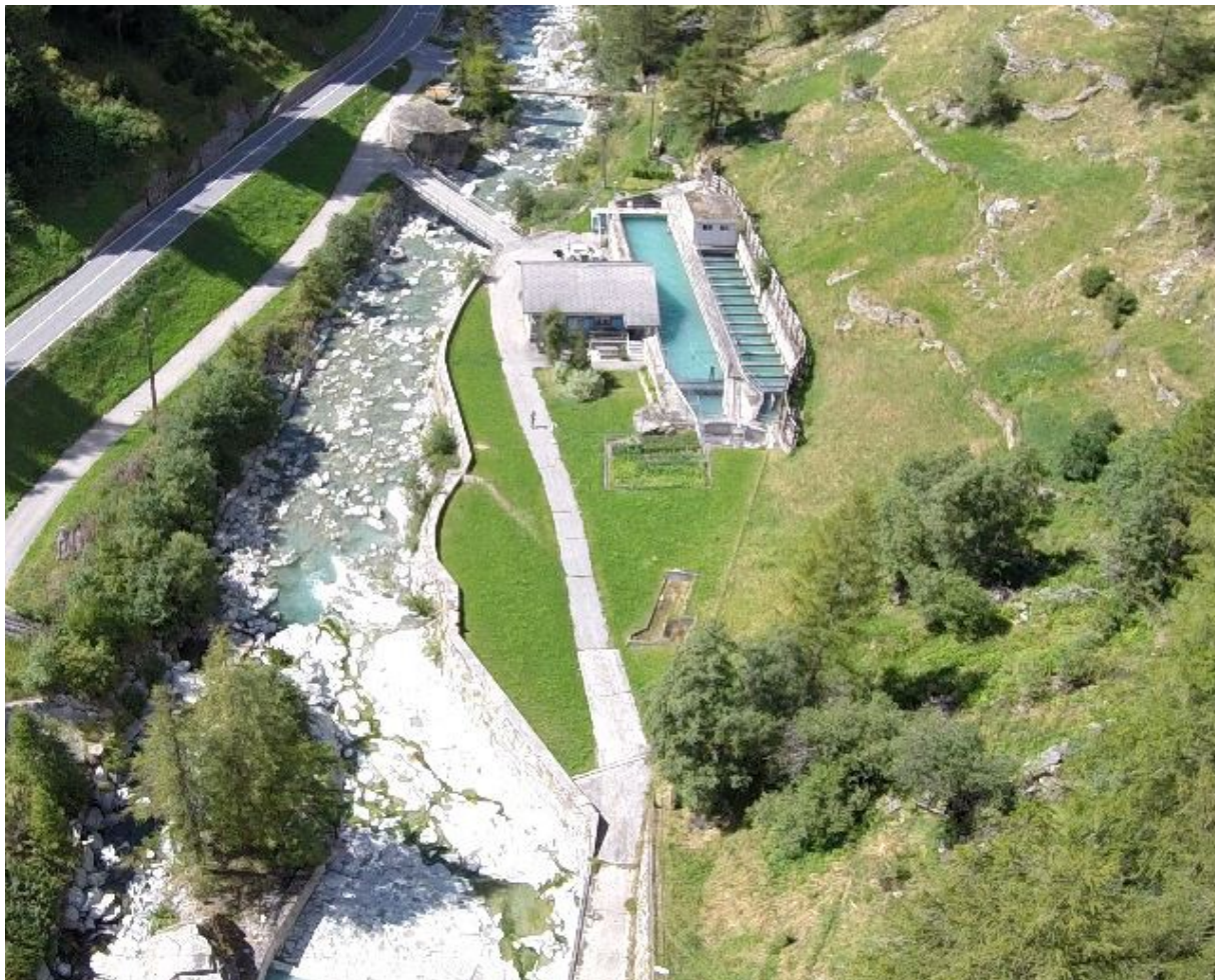
Before water can drive turbines, it must pass through desanding facilities: a plant near Saas-Balen in the canton of Valais Source: VAW / ETHZ
