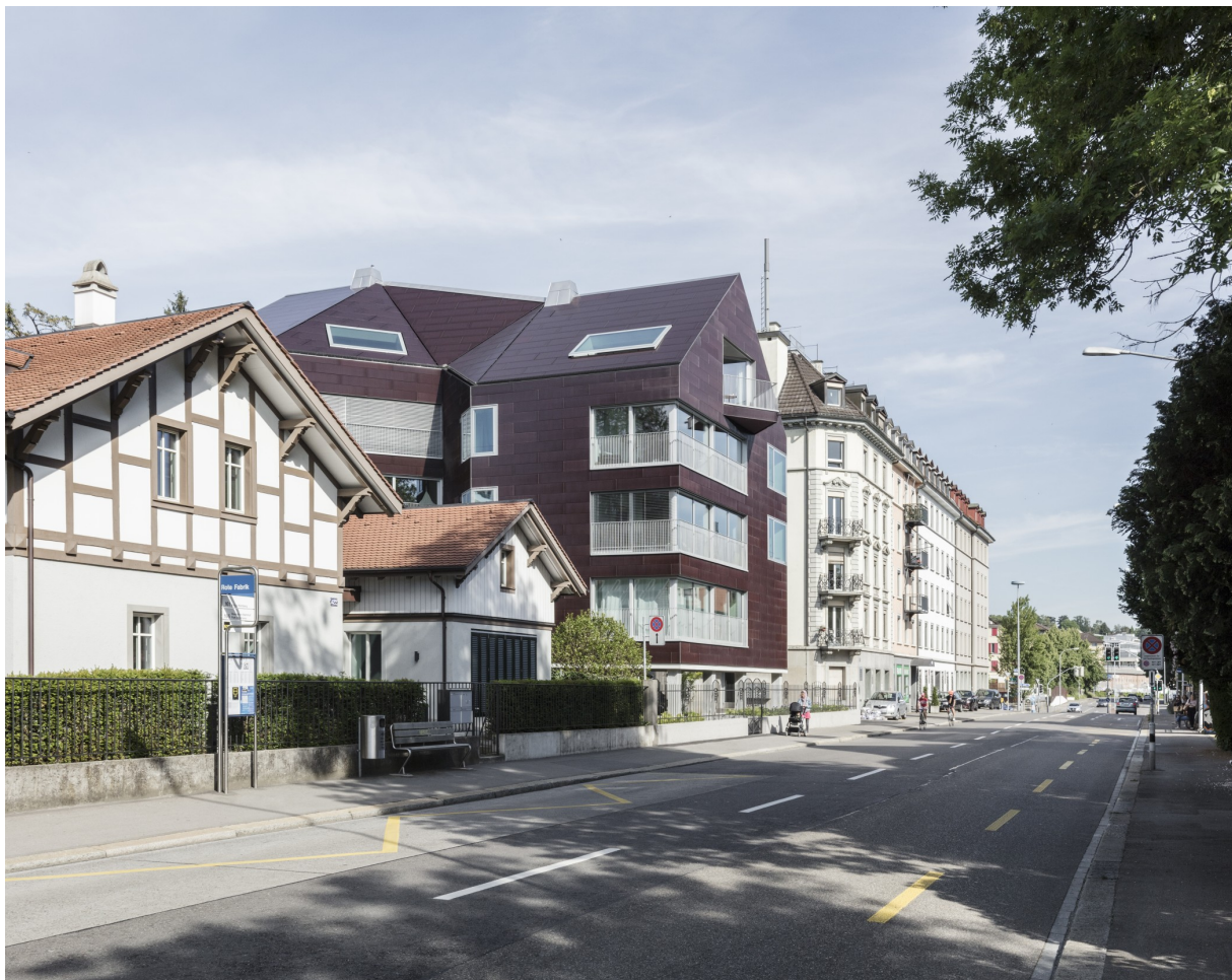
Good demonstration projects, such as this building in Zurich with an active facade, are needed in order to enthuse the population about photovoltaic systems on buildings. Source: Beat Bühler
