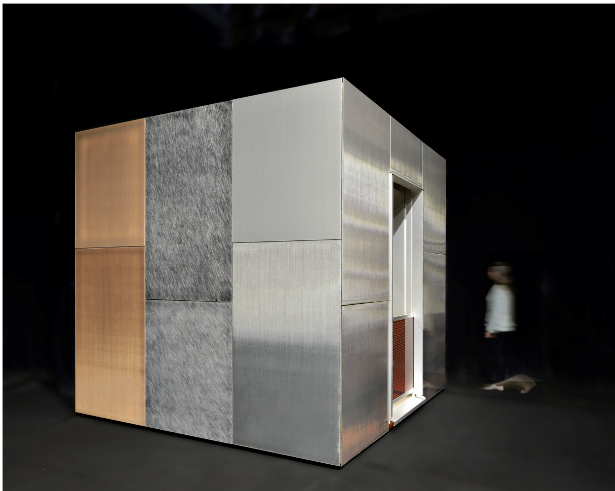
The demonstration cube shows the aesthetic and technical possibilities of new facade elements with integrated photovoltaics in their original scale. Source: Final report Perret-Aebi
