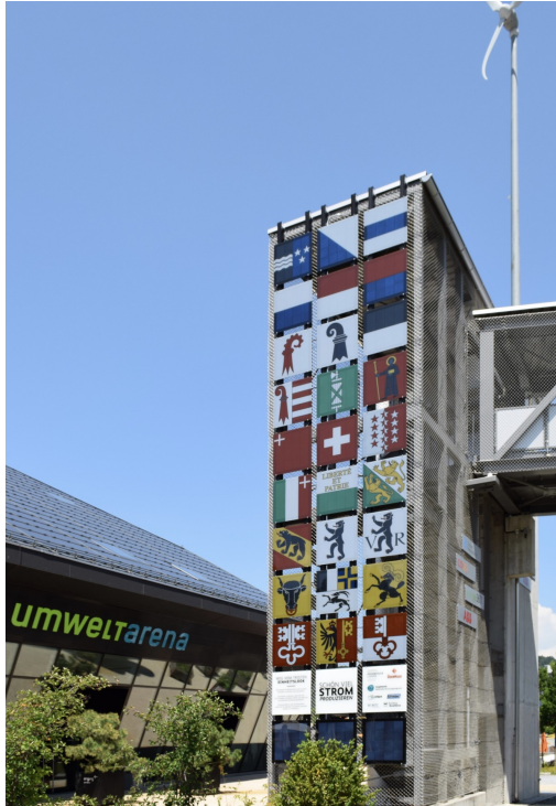
PV modules with the cantonal coats of arms on the stair tower of the Umwelt Arena Schweiz in Spreitenbach. Stephen Wittkopf
